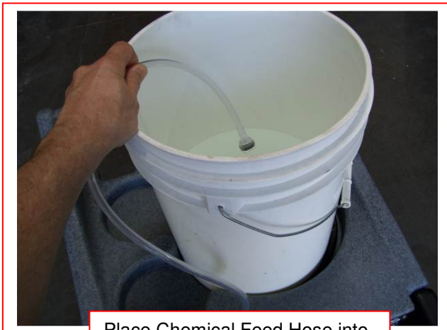
Place Chemical Feed Hose into Rinse Solution
